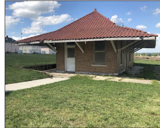
17 Train Depot (Building 105)
