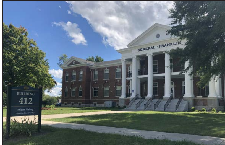
8 "General Franklin" Barracks (Building 412)
