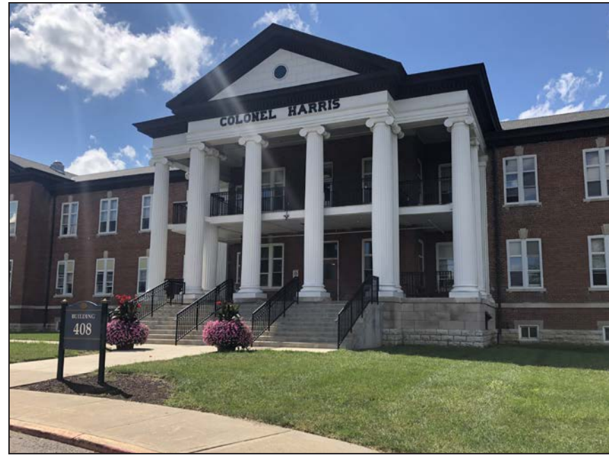
10 "Colonel Harris" Barracks (Building 408)
